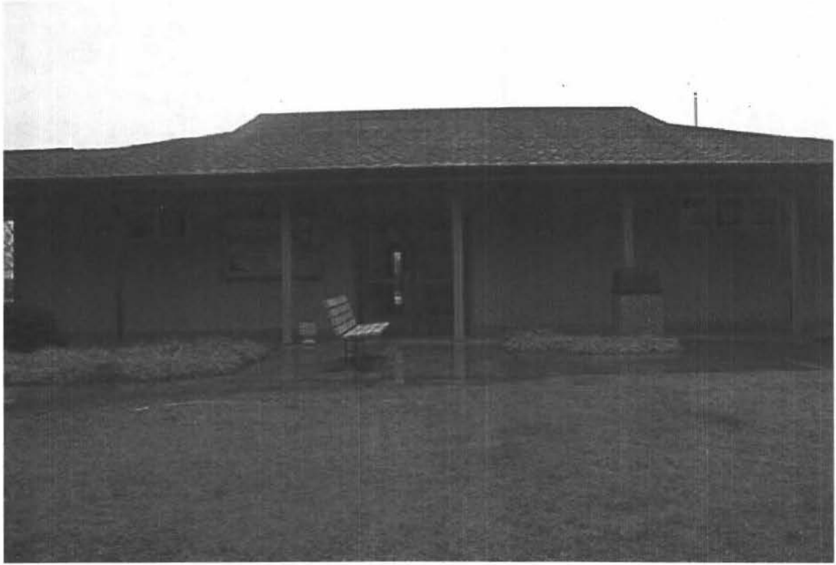
RESTROOM BUILDING FA# 15-04-02
